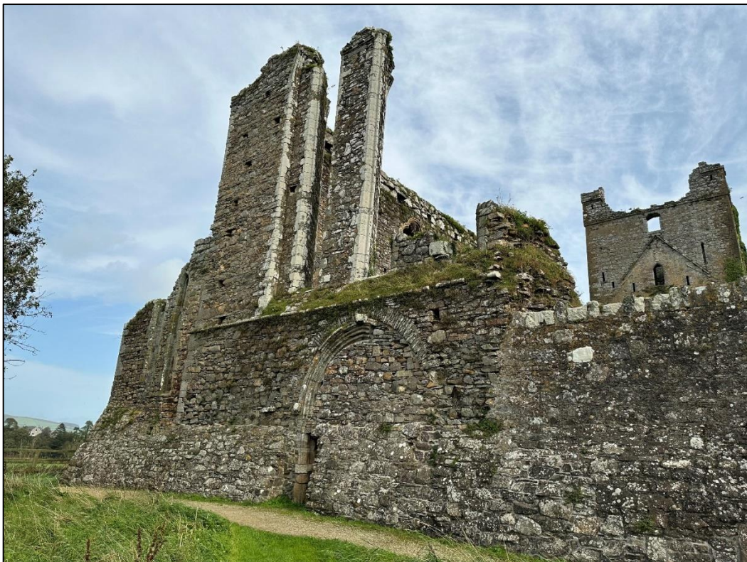
Plate 9 The western elevation of the monastery showing the former doorway into the nave
