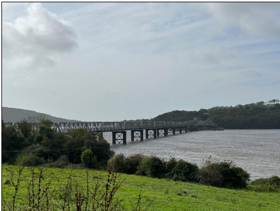
Plate 1 The Barrow Bridge located to the west of the power plant
