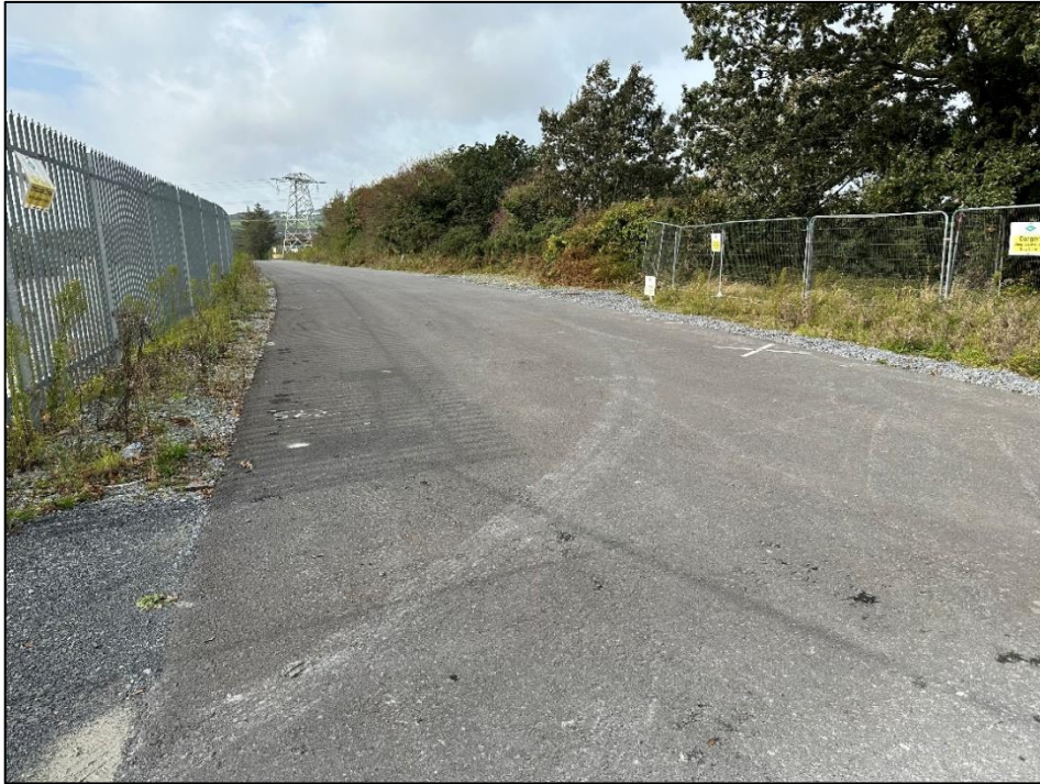
Plate 5 Cable route looking west
