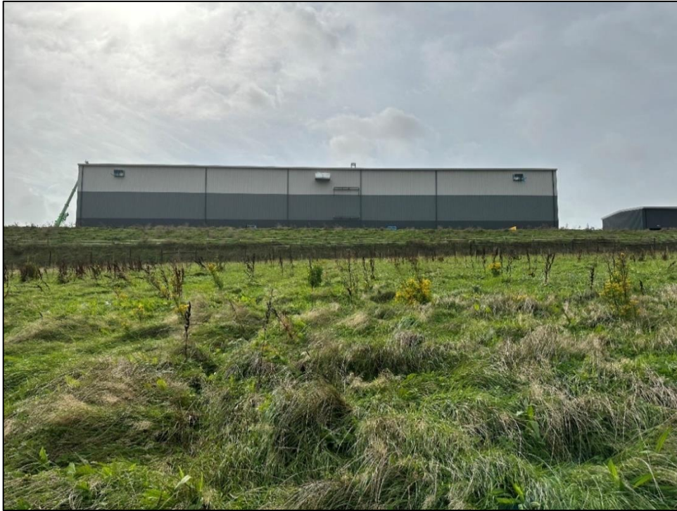
Plate 3 View to the north and the under-construction generator site
