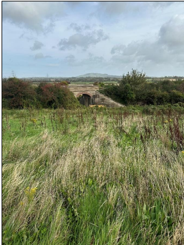
Plate 4 View towards the railway bridge located outside the northeast corner of the site
