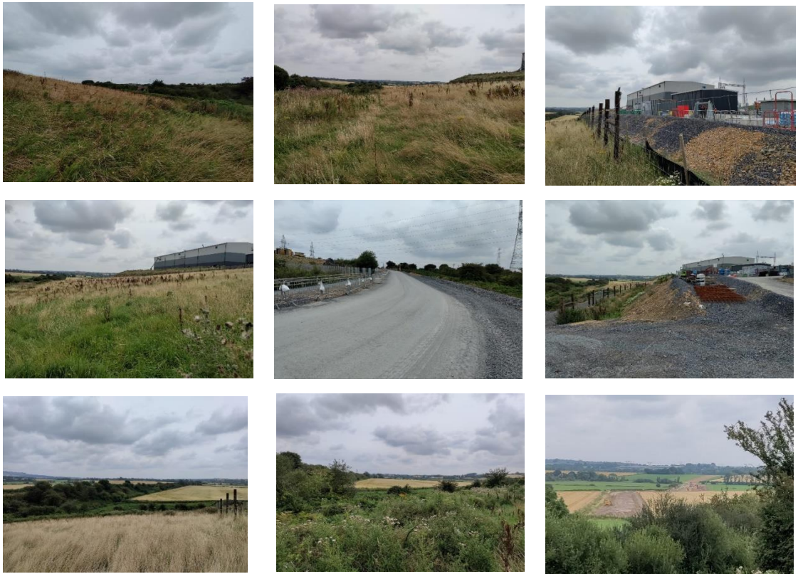
Figure 5 – Site visit photographs – Lands at Great Island, Kilmokea, Co. Wexford
