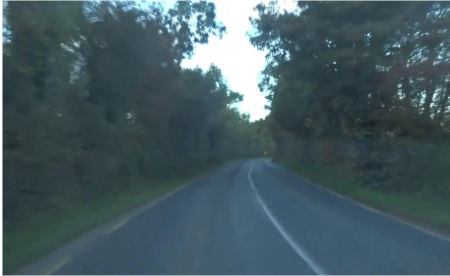
Photo 3: R733 (adjacent to the L4033 junction)
