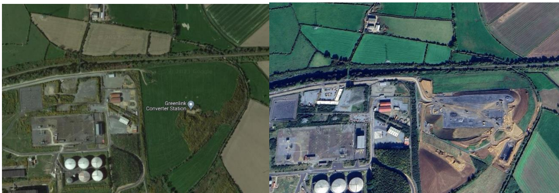
Figure 5-1: Original site (left image) located to east of Great Island power station compared to more recent works (right image)
