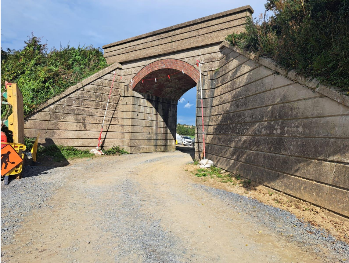
Plate 5-1: Bridge to north-west of site.
